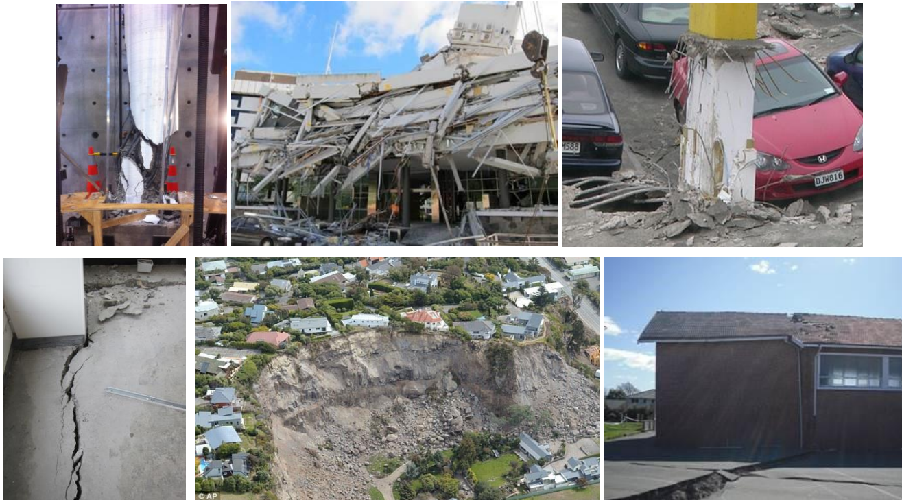
Figure 7: Severe Structural Weaknesses (SSWs): a) non-ductile reinforced concrete column with axial-shear failure; b) Pyne Gould Corp building collapse in Christchurch – non-ductile single core wall without redundancy c) flat-slab punching shear failure d) diaphragm detachment failure e) loss of building platform due to mass slope failure f) splitting and near-collapse unreinforced masonry church due to liquefaction and lateral spreading.
