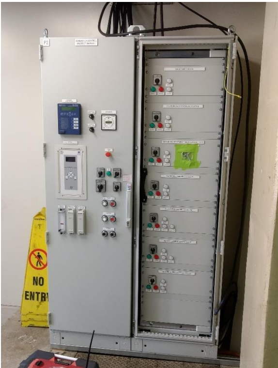
Figure 8 Switchboard and Turbine Alternator Remote Control Panel
