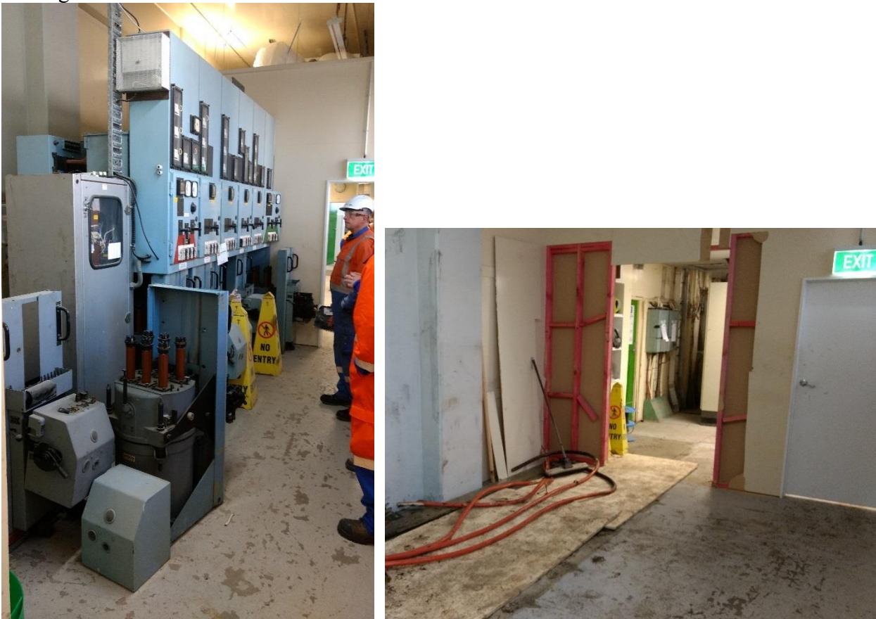
Figure 4 Demolition of the Old Switchboard, before and after
