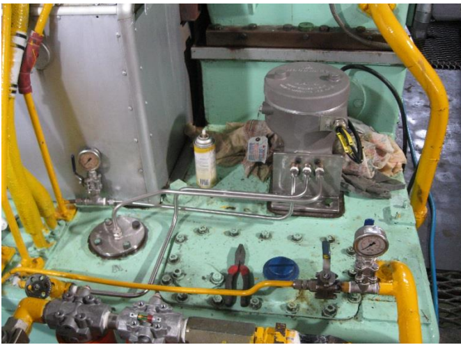
Figure 12 Electro-Hydraulic Interface Installation
