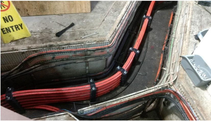
Figure 6 New HV cables and cable clamps
