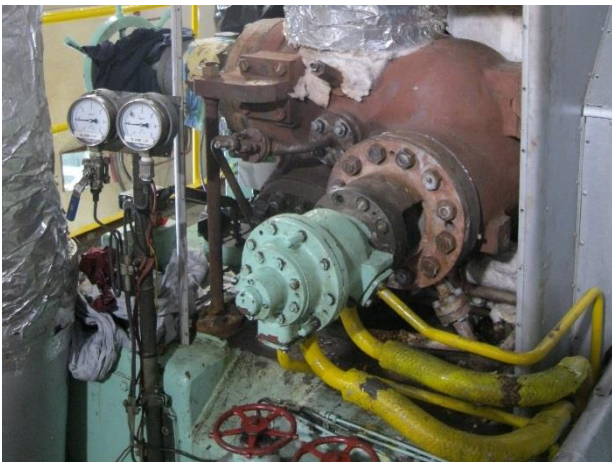
Figure 10 Pilot Actuated Hydraulic Servo
