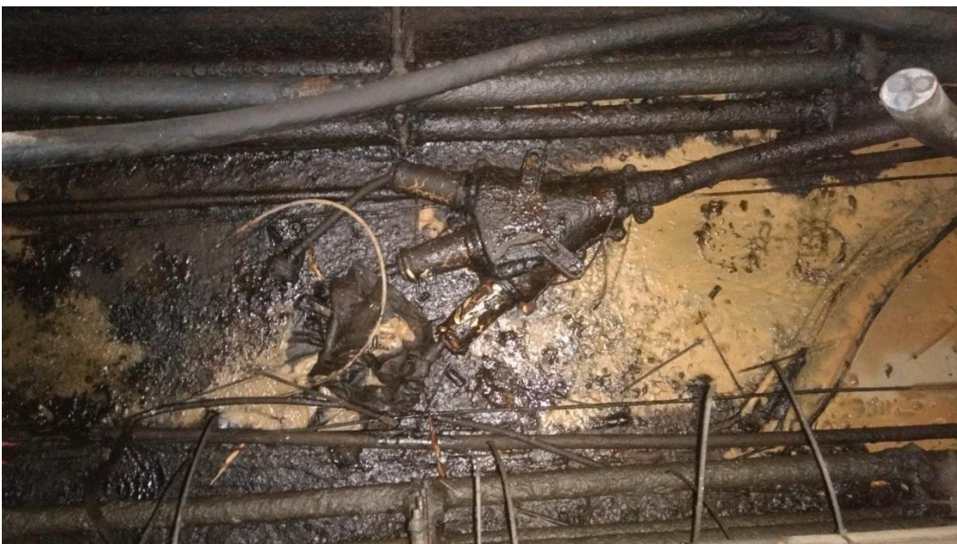
Figure 5 Cable trench before cleanout
