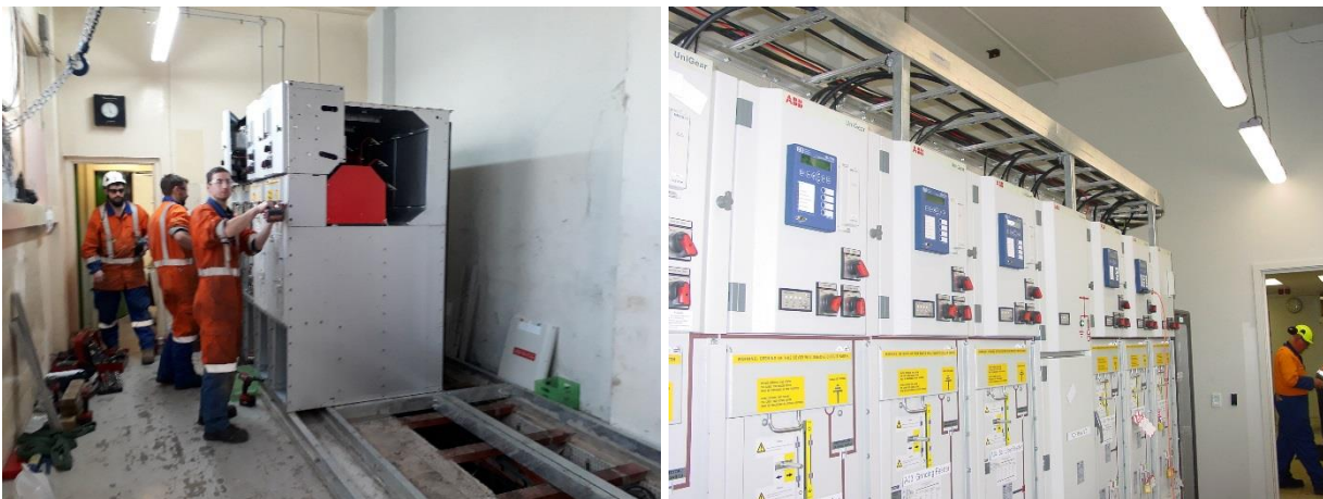
Figure 7 Switchboard installation and as commissioned
