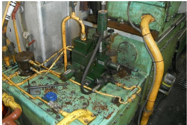
Figure 11 Askania Steam Pressure Regulator
