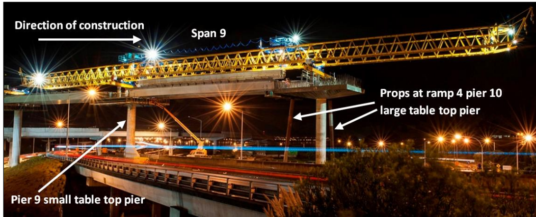
Figure 3. Ramp 4 table top spans & props installed at Ramp 4 pier 10
