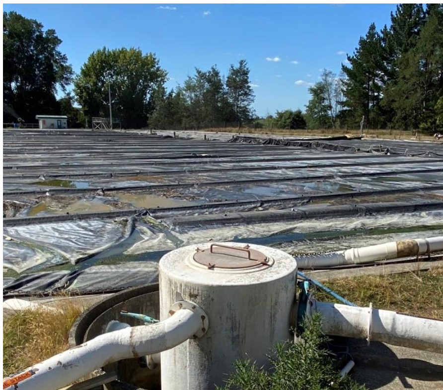
Figure 5: Fonterra's Tirau Anaerobic Lagoon Digestion Plant
