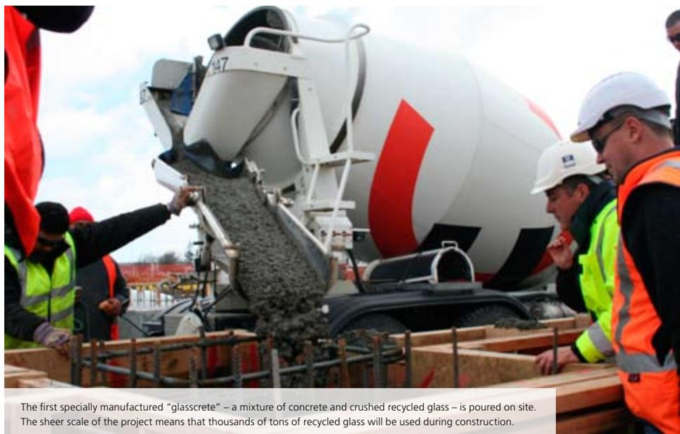
The first specially manufactured "glasscrete" – a mixture of concrete and crushed recycled glass – is poured on site. The sheer scale of the project means that thousands of tons of recycled glass will be used during construction.
