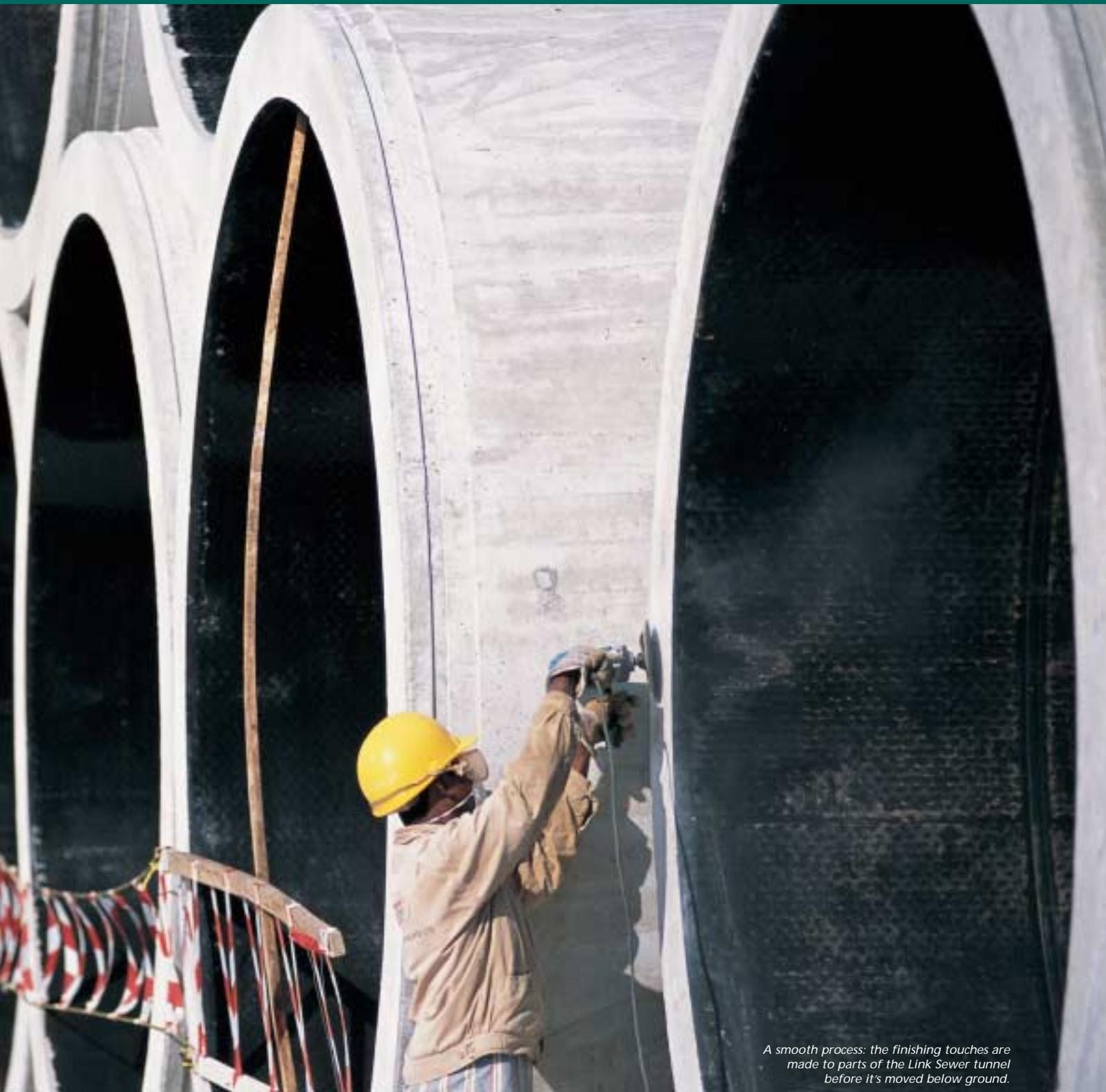
*A smooth process: the finishing touches are made to parts of the Link Sewer tunnel before it's moved below ground.*
