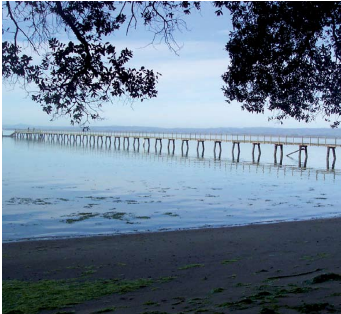
Kauri Point Wharf (Western Bay of Plenty) structure
