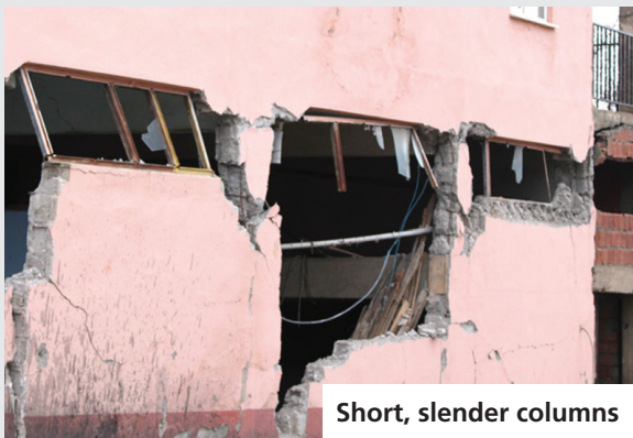
Masonry infill walls
